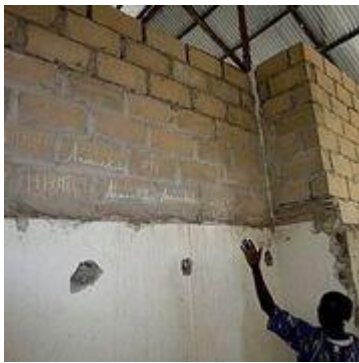
Project 4 – Verhoging muren
